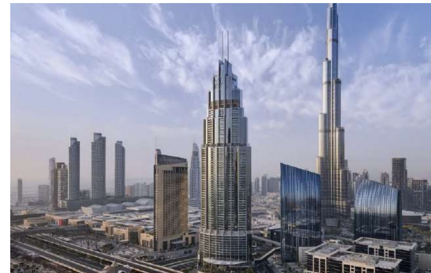
Address Boulevard 11th Floor Luxury Suites Renovation
