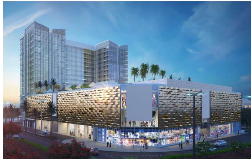
Al Mamzar Byblos Hotel, Guestroom MEP Works
