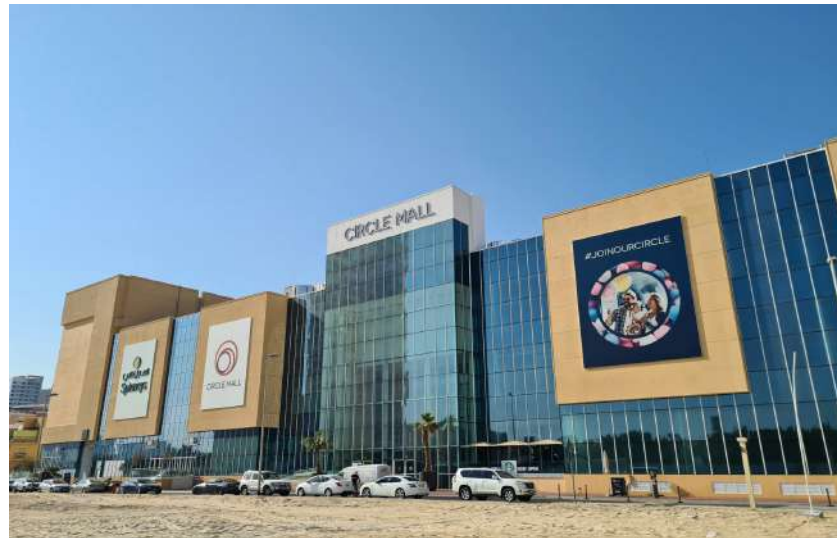
Circle Mall Jumeirah Village Circle, 2nd Floor MEP Works
