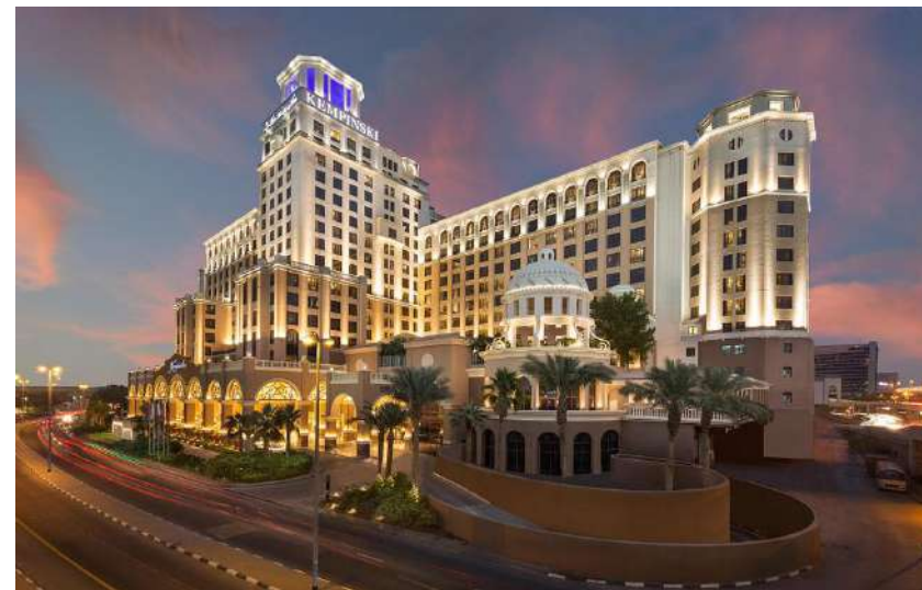
Kempinski Hotel MOE Lightning Protection System
